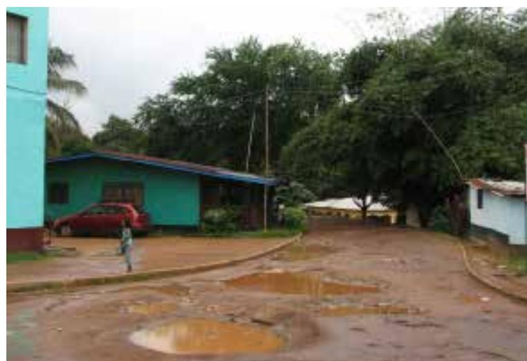
Figure 74. Road in Old Matadi. Note that even metalled roads in government-developed housing areas have little drainage, in one of the wettest countries in the world
