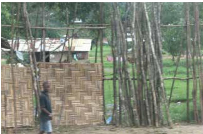
Figure 86. Poles and bamboo mats for construction, Gbarnga
