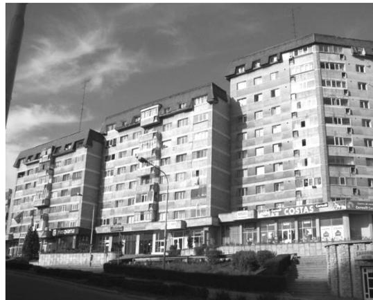
The 1980s: Blocks in prefabricated concrete panels
